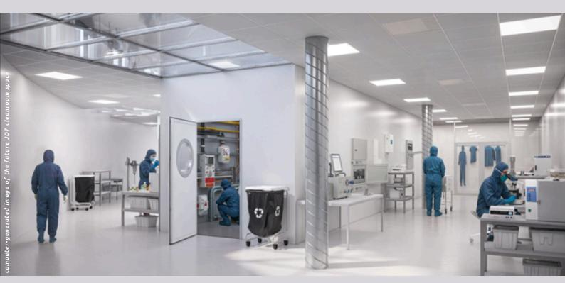
JD7's cleanroom infrastructure complies with ISO 14644-1 Class 5 standards (equivalent to Class 100 under the former US FED STD 209E). This classification ensures extremely low airborne particulate levels and highly stable environmental conditions, essential for operations at micro- and nanoscale.
